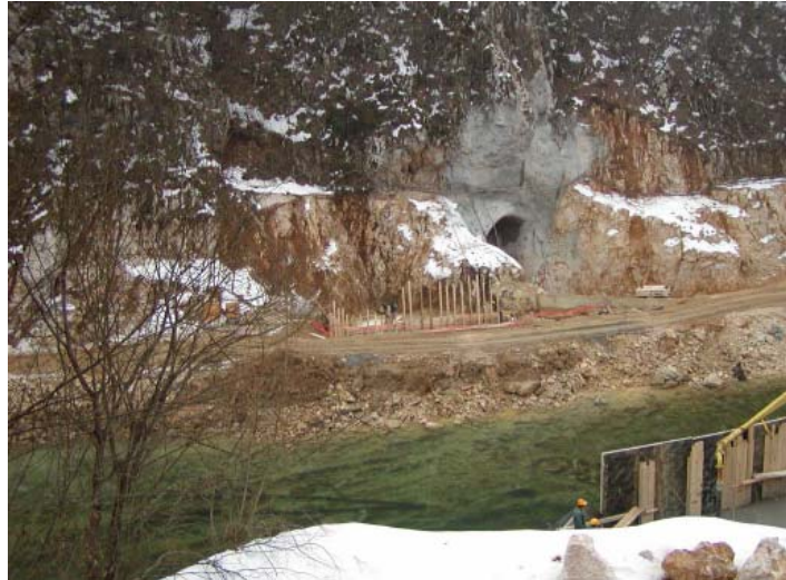
HE Lešće – ulaz u obilazni tunel
